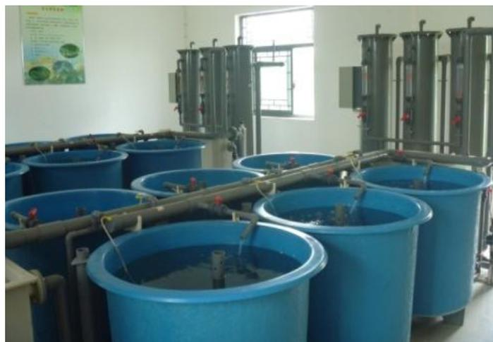
**Fig.2** Indoor water recirculation system
